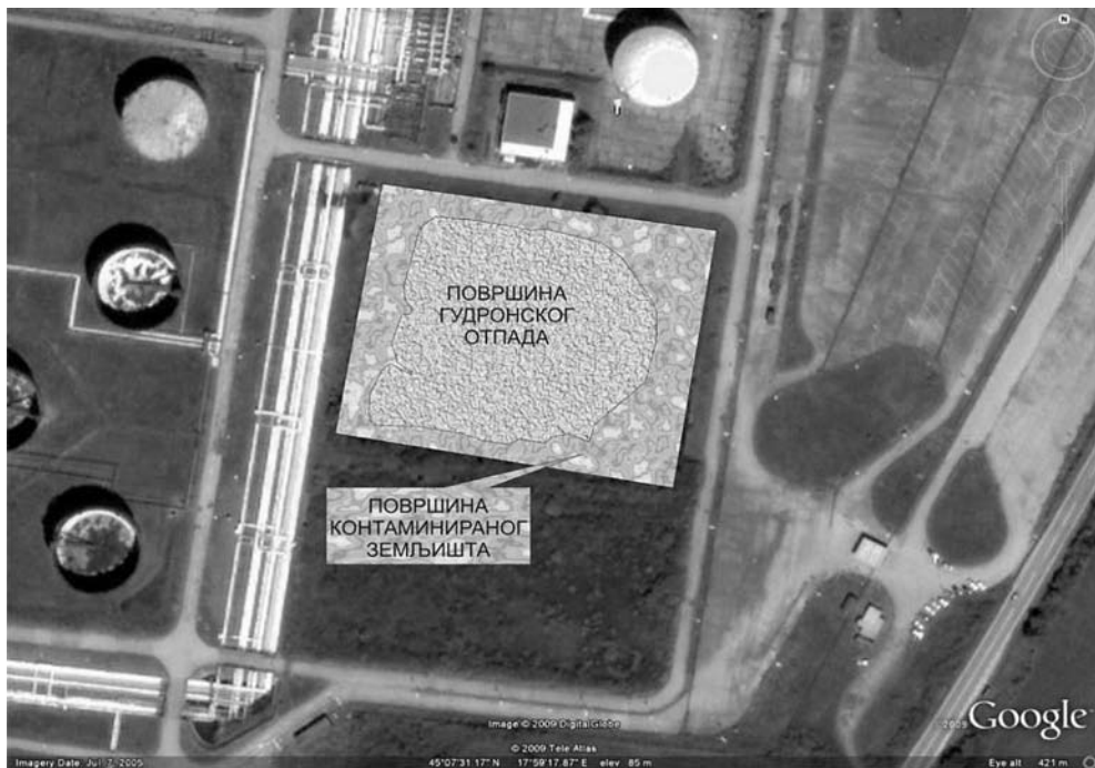
Figure 3.: The disposition of areas at acid tar sludge landfill in Oil Refinery in Bosanski Brod.
