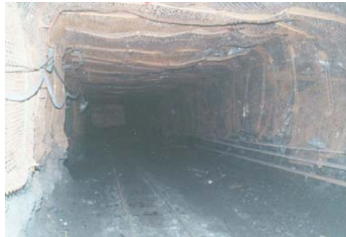
Figure 2.: In-situ support state of solid roadway in 7401 coalface.
