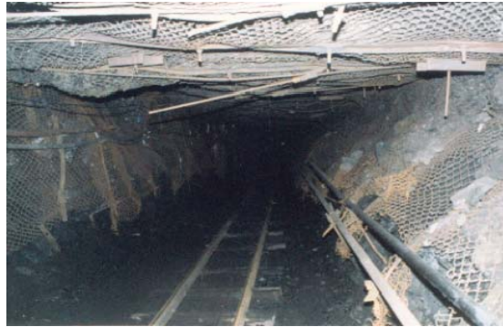
Figure 6.: In-situ support state of entry driven head-on adjacent advancing coalface (width of pillar, 4m).
