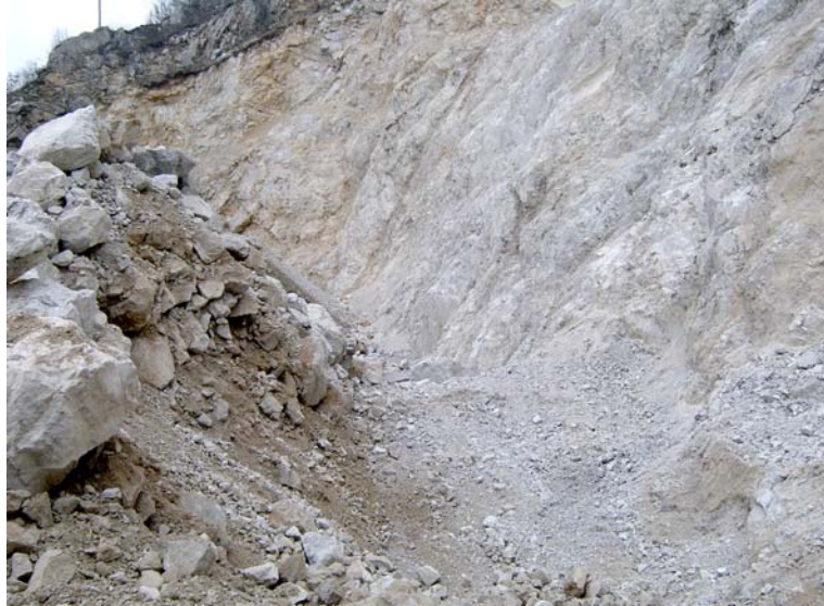
Figure 6.: Embankment and channel between rock quarry and wastewater collectors. Total height of channel and embankment is 8 m.
