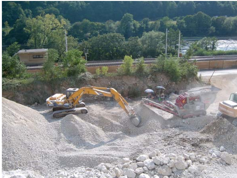
Figure 2.: Embankment between rock quarry and the road.
